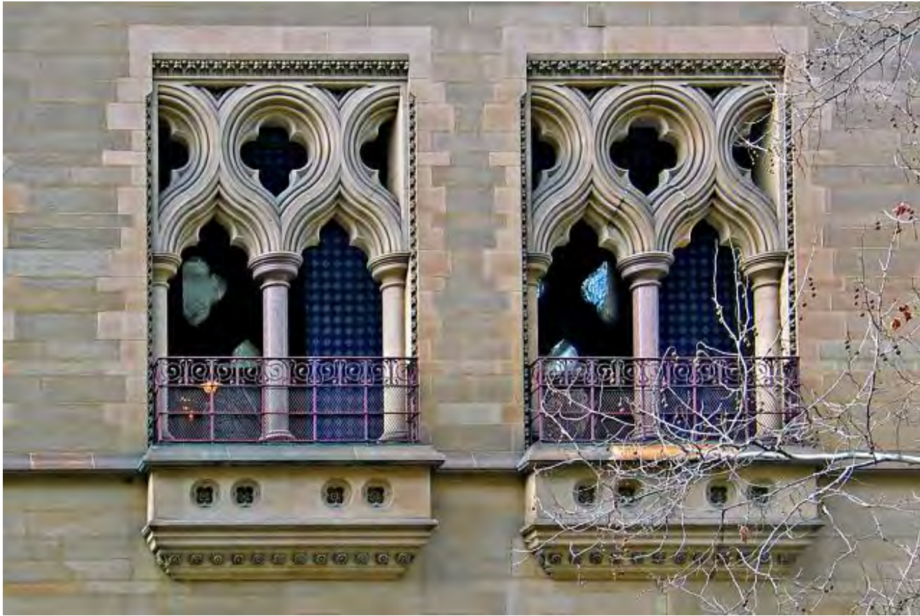
William WARDELL 1824-1899, Gothic ANZ Bank, Window detail, Queens St Elevation, 1883
